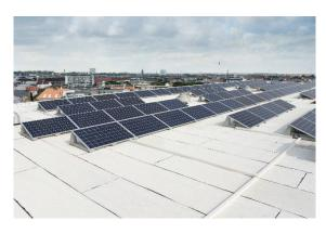
In most policies, the installation of PV systems is considered a relevant change to the building which must be reported to the building insurer. Movable PV installations placed on the roof are not always regarded as part of the property and therefore may not be covered by the home insurance. In order to limit the cost of damage caused by fires in PV installations on roofs, insurers and insurance brokers are incited to adjust their policy conditions.
